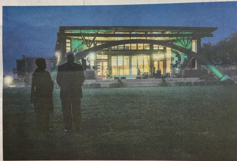
>TE Kura Whare in Taneatua is one of 14 buildings in the world to have reached a no impact standard.
