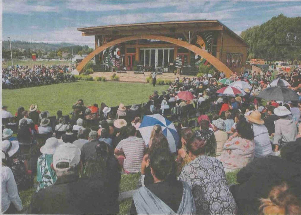
NO IMPACT: Te Kura Whare in Tanetua is one of 14 buildings in the world to have reached a no impact standard.
